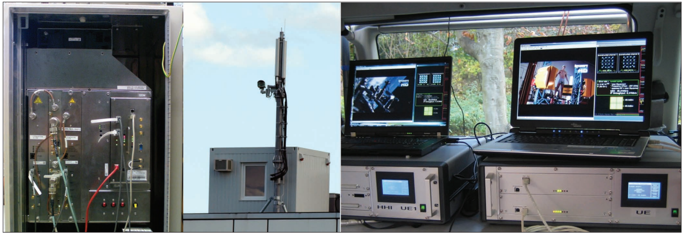
Figure 4. Testbed hardware. Left: base station hardware for one sector. Center: antenna setup on top of the TUB main building. Right: test terminals in the measurement van.
